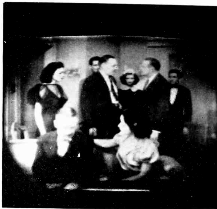
Fig. 10—Images photographed directly from the mirror of the receiver, during the telecast of "The Donovan Affair" from the NBC transmitter. Exposures 1/10th second, at f/4.5 , Agfa Superpan Press, enlargement about four times
