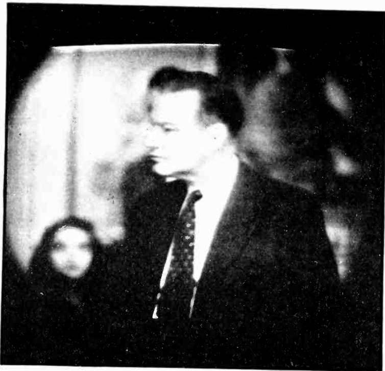
Fig. 10—Images photographed directly from the mirror of the receiver, during the telecast of "The Donovan Affair" from the NBC transmitter. Exposures 1/10th second, at f/4.5 , Agfa Superpan Press, enlargement about four times
